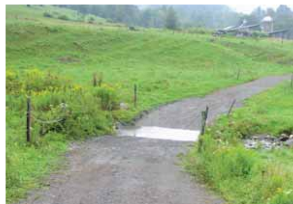
Geotextile fabric is placed under stone (above) to construct this ford-type stream crossing on an organic dairy farm in Guilford, VT. (Below) Completed stream crossing ready for use.
