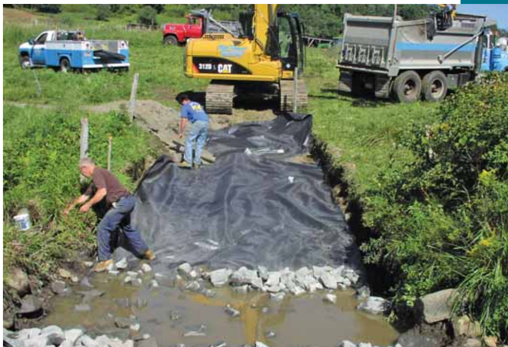
Geotextile fabric is placed under stone (above) to construct this ford-type stream crossing on an organic dairy farm in Guilford, VT. (Below) Completed stream crossing ready for use.
