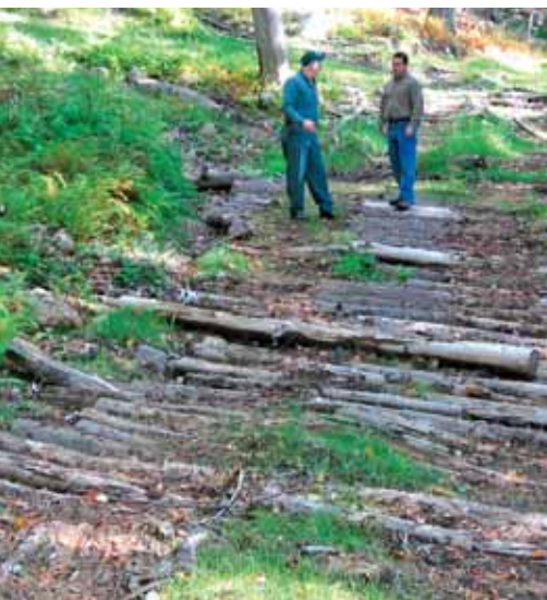
Log corduroy help create access over wet areas and provides organic matter to soil.
