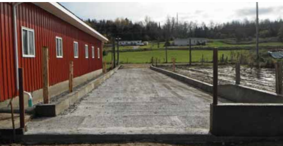
Gutters and a concrete use area ensure that water is properly directed away from farmstead.
