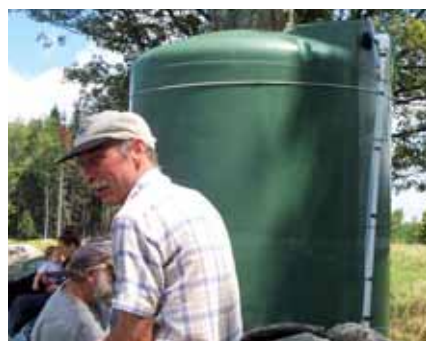
This water storage tank on the Corse Farm in Whitingham is supplied by a solar-powered pump that is located in a nearby spring. Water is then gravity fed from the tank to a system of watering tubs that are located throughout the farms' pastures. This farm is pasture-based and uses a rotational grazing system.
