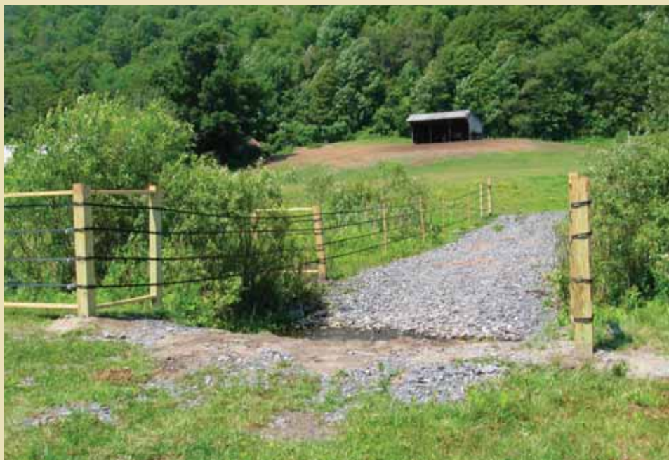
Livestock exclusion fencing and an armored stream crossing on Highbrook Farm, S. Woodstock, VT.
