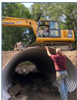
Conservation Districts support healthy aquatic habitats in a number of ways. Essex County NRCD coordinated a culvert replacement on a tributary to the Connecticut River to restore Aquatic Organism Passage, with funding support from U.S Fish & Wildlife.
