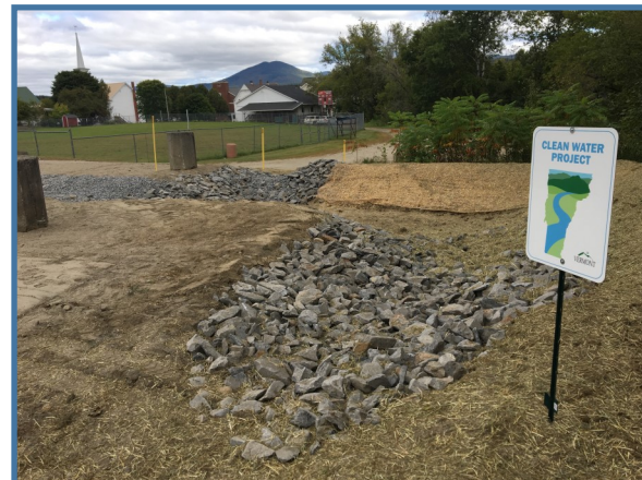
Installation of grassed swales and sediment basins at the Fenton Chester Ice Arena in Lyndon, treating stormwater from a 1.4 acre gravel parking lot to reduce runoff to the stream, coordinated by Caledonia County NRCD and funded by the VT DEC Block grant
