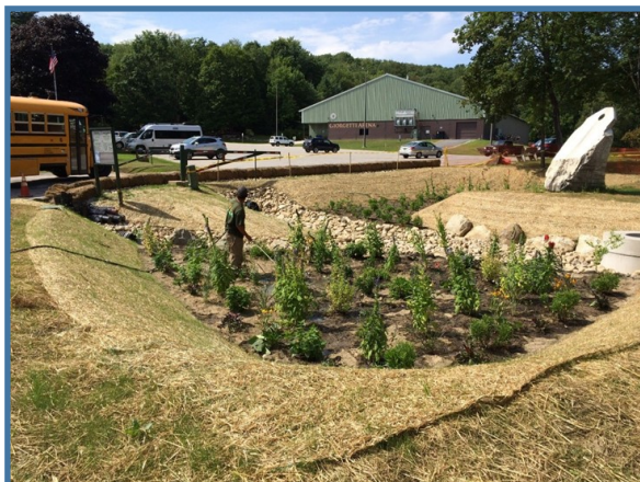
A bioretention basin infiltrating stormwater installed at Georgetti Park in Rutland City, a project identified in the East Creek Watershed Stormwater Master Plan, coordinated by Rutland NRCD and funded by the Ecosystem Restoration Program
