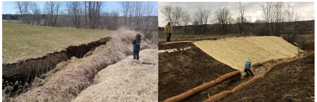
Left, “Before:” A small tributary to the Pike River incised and undercut it’s banks, resulting in a bank failure in April 2018. Right, “In-Progress:” District staff, ECOAmeriCorps members, and EcoSolutions work to install erosion control fabric on the slopes of the banks, which now lie at a more stable angle less prone to failure. We will share an “after” picture once the project has been revegetated next year!
