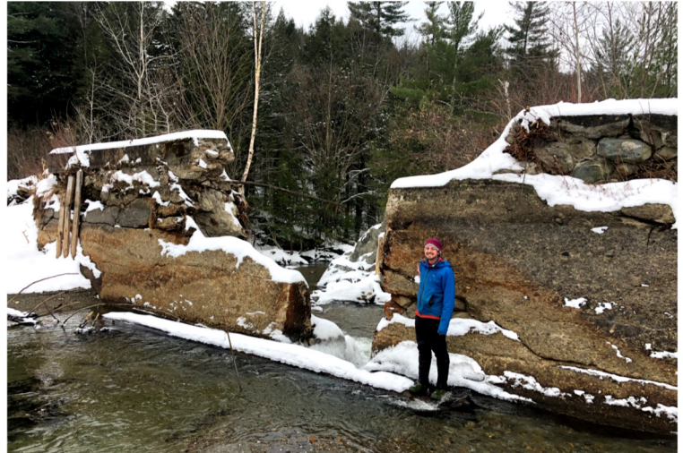
Brodie Haenke stands upstream of the now-breached Johnsons Mill Dam in Bakersfield. The project will remove sufficient concrete to allow brook trout to pass through the old dam and will remove impounded sediment behind the dam.
