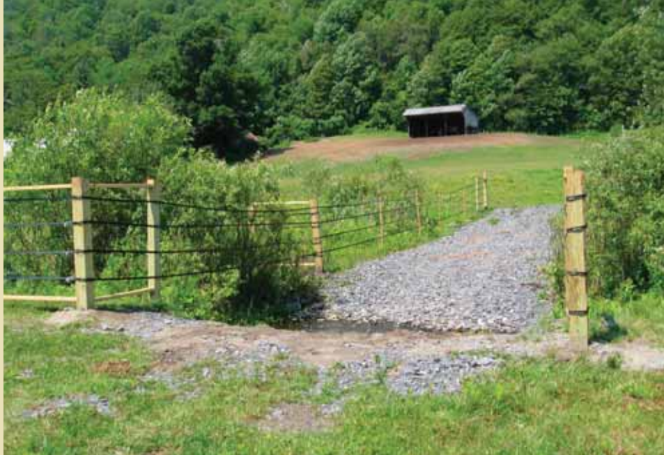
Livestock exclusion fencing and an armored stream crossing on Highbrook Farm, S. Woodstock, VT.
