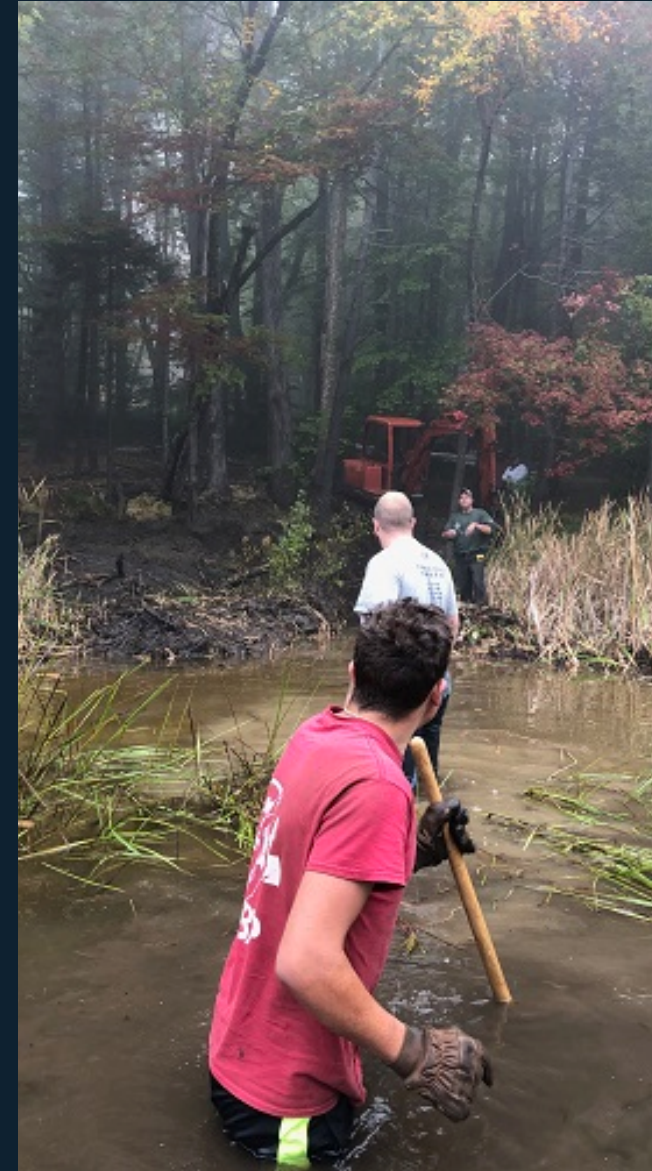
Firefighters in Townshend ensuring the dry hydrant intake is properly placed
