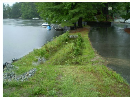
Vegetative swale with rock check dam treats 98% of road runoff to lake
